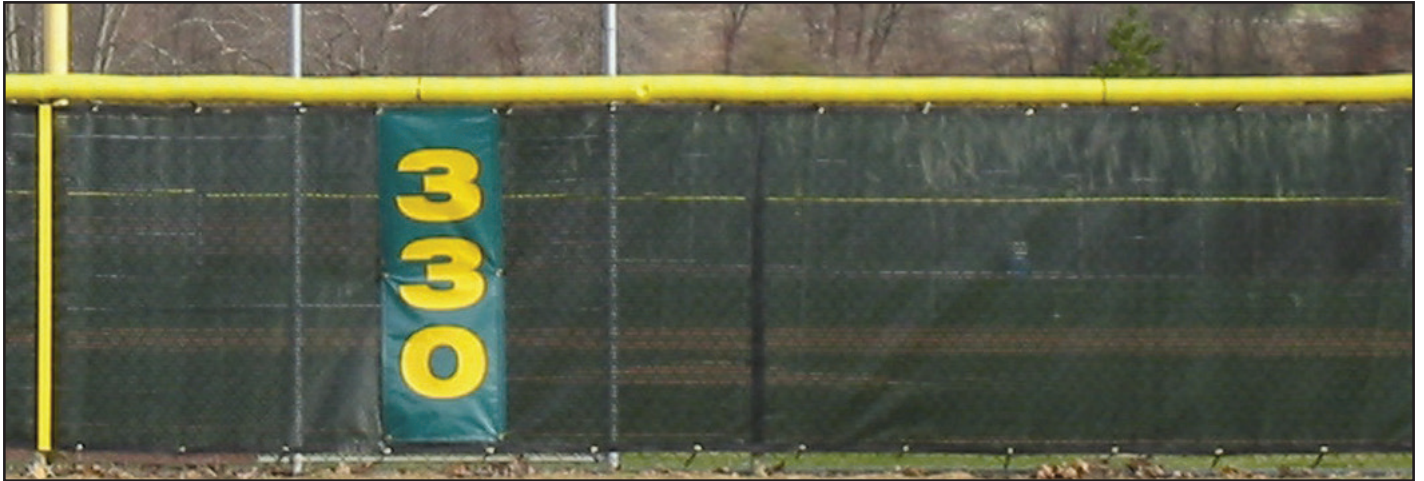
Windscreen properly installed
